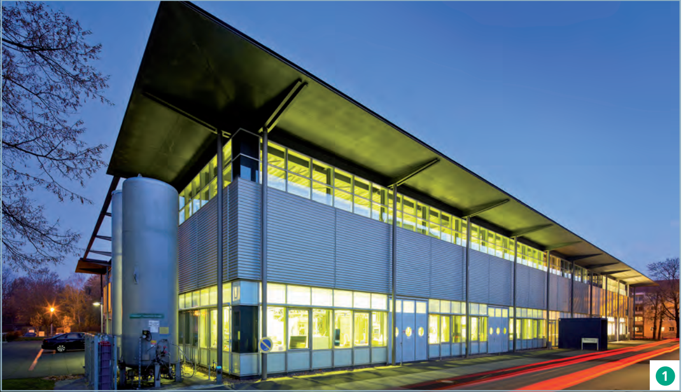
Institute Center Dresden, Fraunhofer FEP Technology Center, Winterbergstraße
